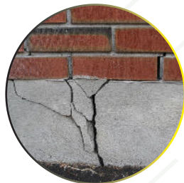
FOUNDATION CRACKS
